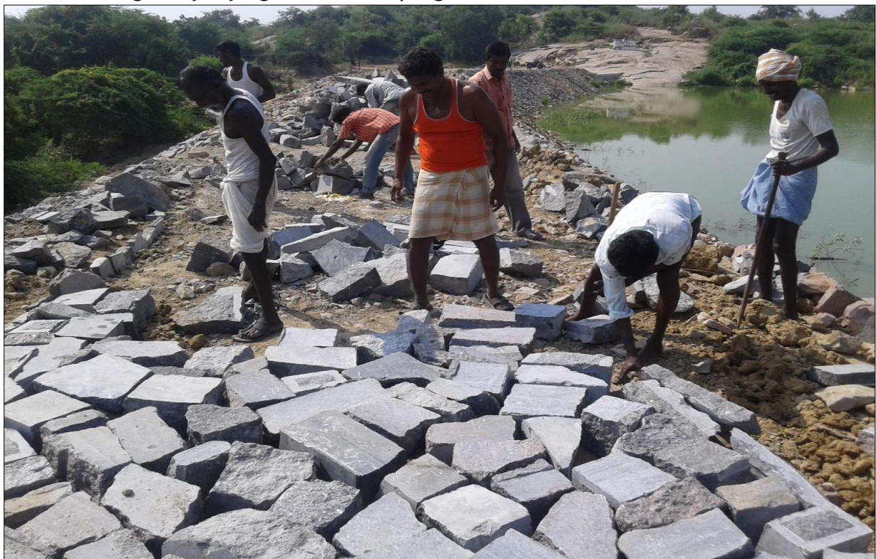
28. Carriage way laying work under progress
