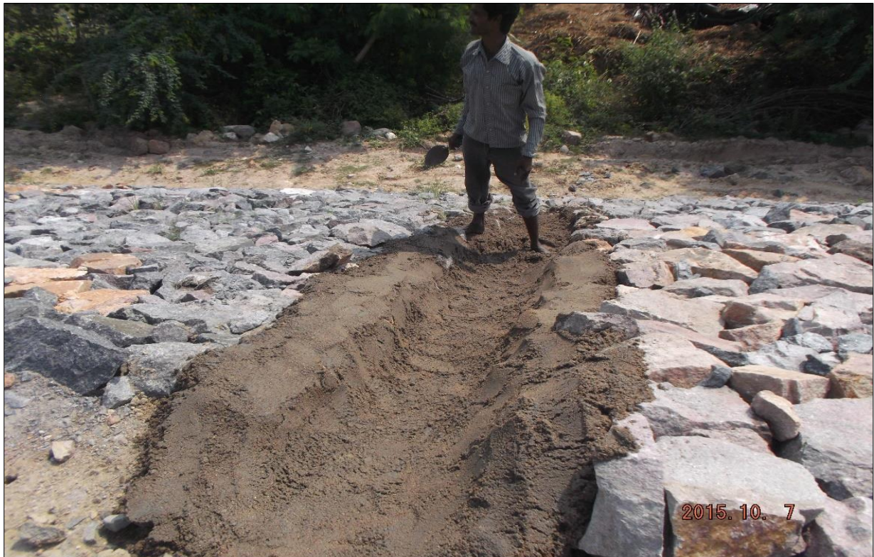
27. Bund side drains under progress
