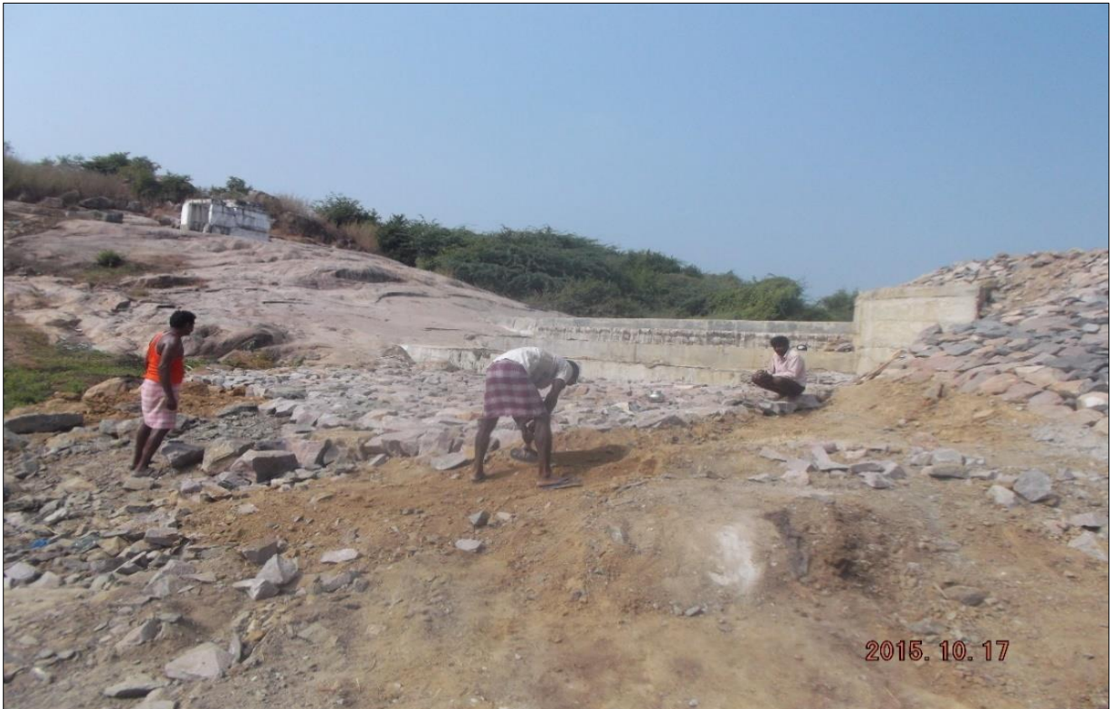
29. Cut of wall pitching work under progress at weir D/S side
